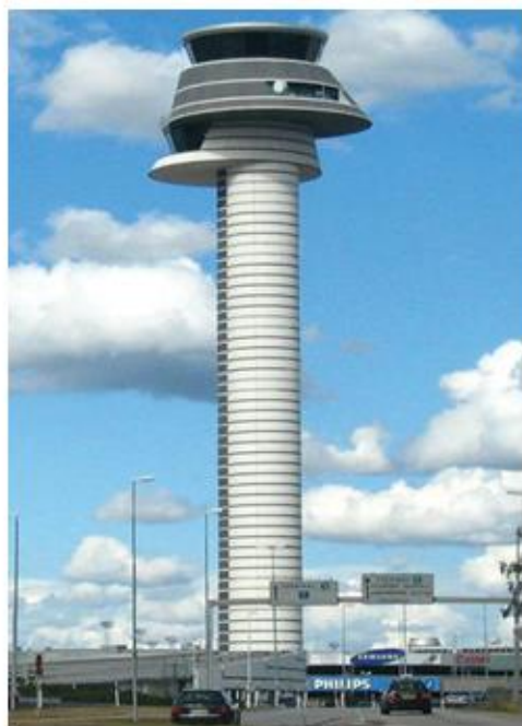
Figure I.2. Arlanda Airport Control Tower Stockholm, Sweden [4]
