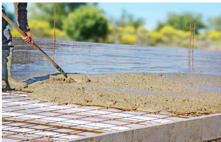
Figure I.1. Application de béton fluide (guide de béton.com/image).
