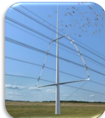
Fig I.11: Pylône monomode Roseau
