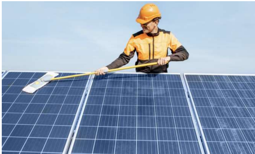
Figure II.22: Image montrant le processus de nettoyage manuel
