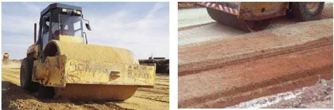
Figure II.8. Types de compactage de surface. [12]
