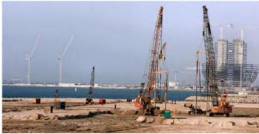
Figure.II.10 Vibrocompactage.[12]
