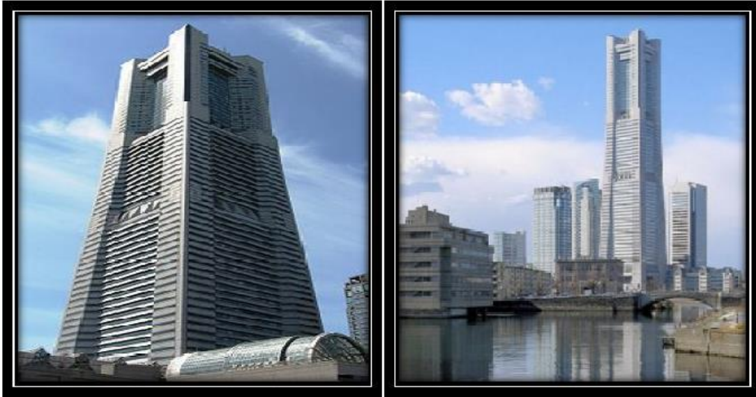
Figure I-9: La tour Landmark Tower (tokyo). [41]
