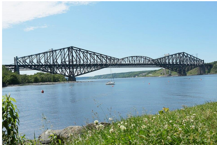
Fig 1.20 Quebec Bridge (Canada) (Cantilever Bridge)
