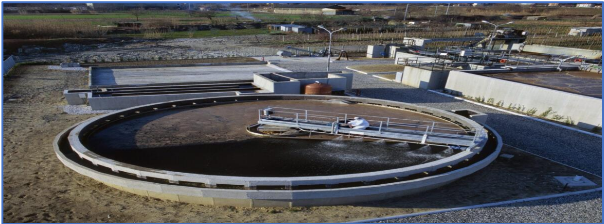
FIGURE 1: BASSIN A BOUES ACTIVE (STEP BBA)
