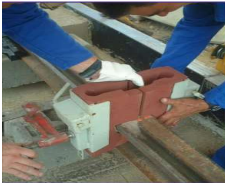
Figure II.6 : Pose du moule
