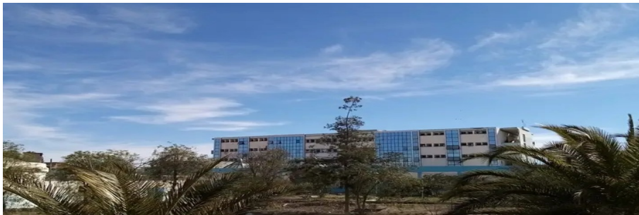
FIGURE 3.1 – Hôpital Bouzidi Lakhdar
