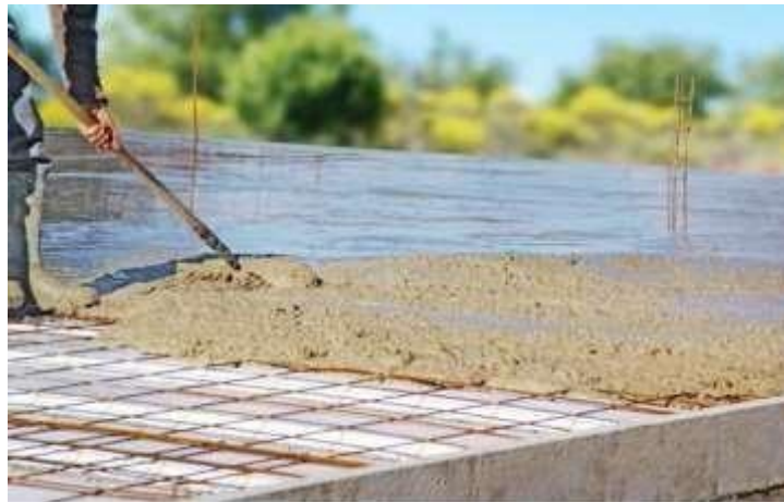
Figure I.1 Application de béton fluide [1]
