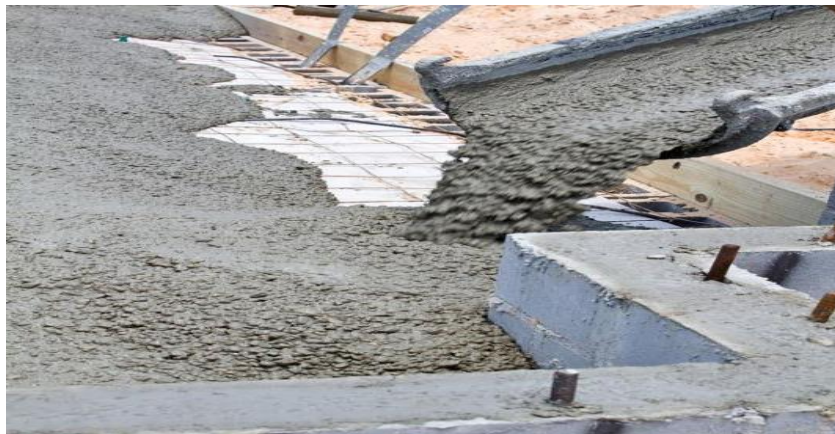
Figure I.1. Application de béton fluide [2].
