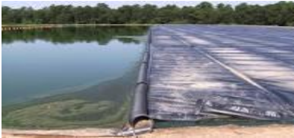
Figure. 2- Les couvertures continues flottantes
