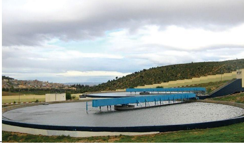
Figure 4: Station d'épuration (site web) [24]
