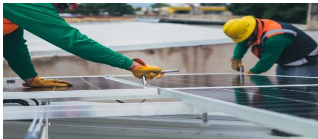
Figure 11: Construction steps of photovoltaic
