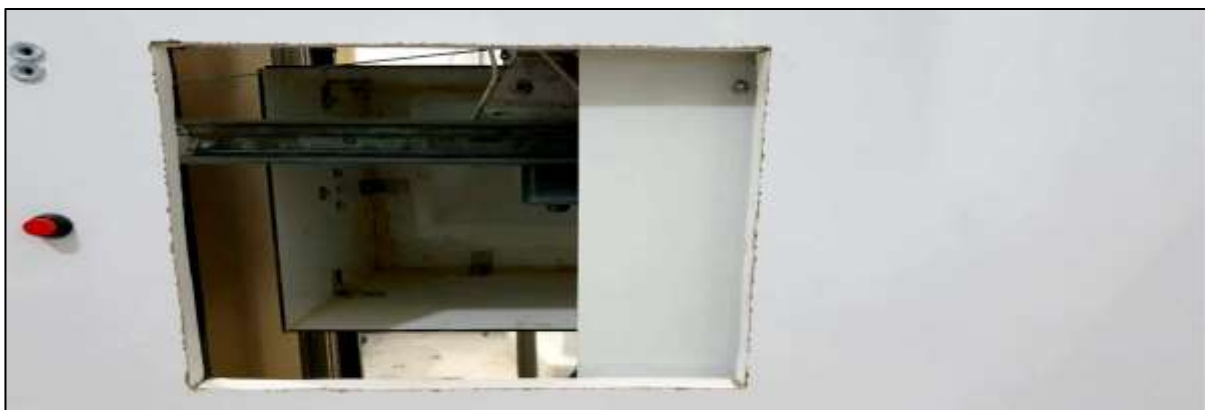
Figure III.19. real picture of opening the 1 st floor door
