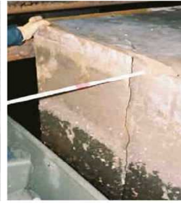
Figure 5.II.1: Fissure.
