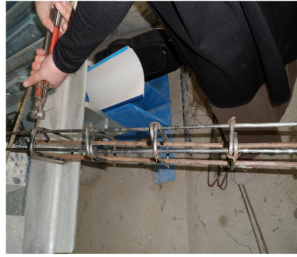
Figure 4.III.2 : Couture d'armature.
