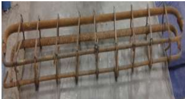
Figure 5.III.2: Ferrailage final de la poutre.
