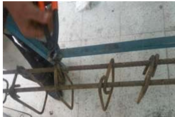
Figure 4.III.2 : Couture d'armature
