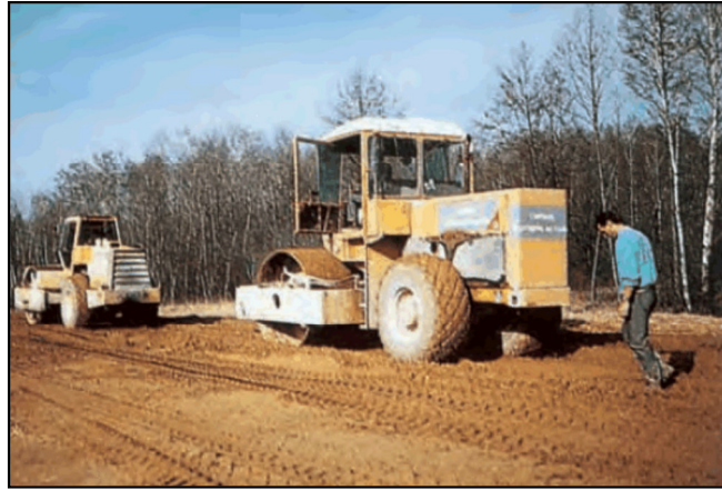
Figure III.6 : Compactage [7].
